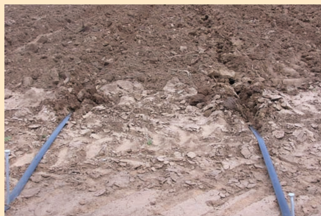
Newly-installed subsurface drip irrigation tubing
