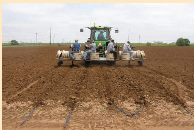
Installing subsurface drip irrigation using a tractor
