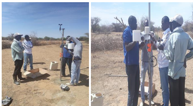
Installation of weather station in the Sanente village
